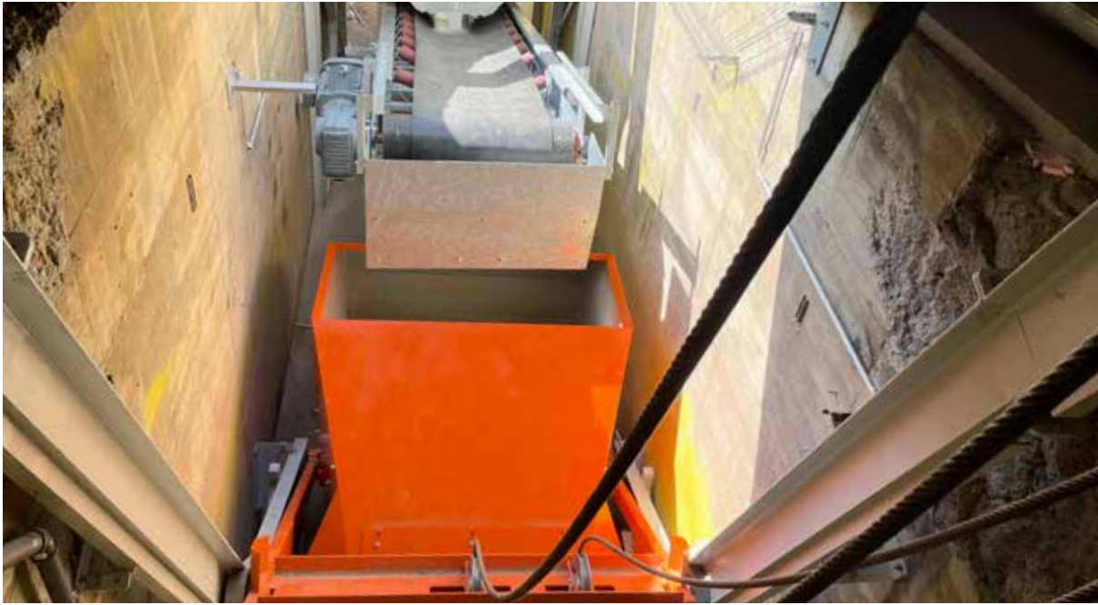
Skip hoist to the mixer with fall protection in operation
