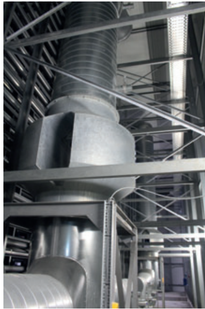
The entire interior air is recirculated by three main fans arranged laterally
