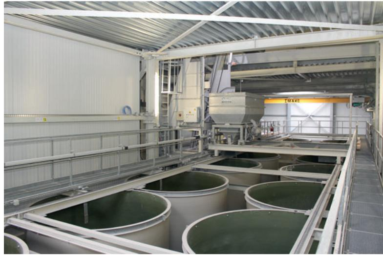
Aggregate transfer to a mobile bucket that can travel in 2 directions takes place upon arrival at the upper level.
